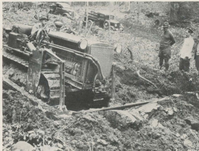
C.C.C. Operating Diesel Trail Builder
