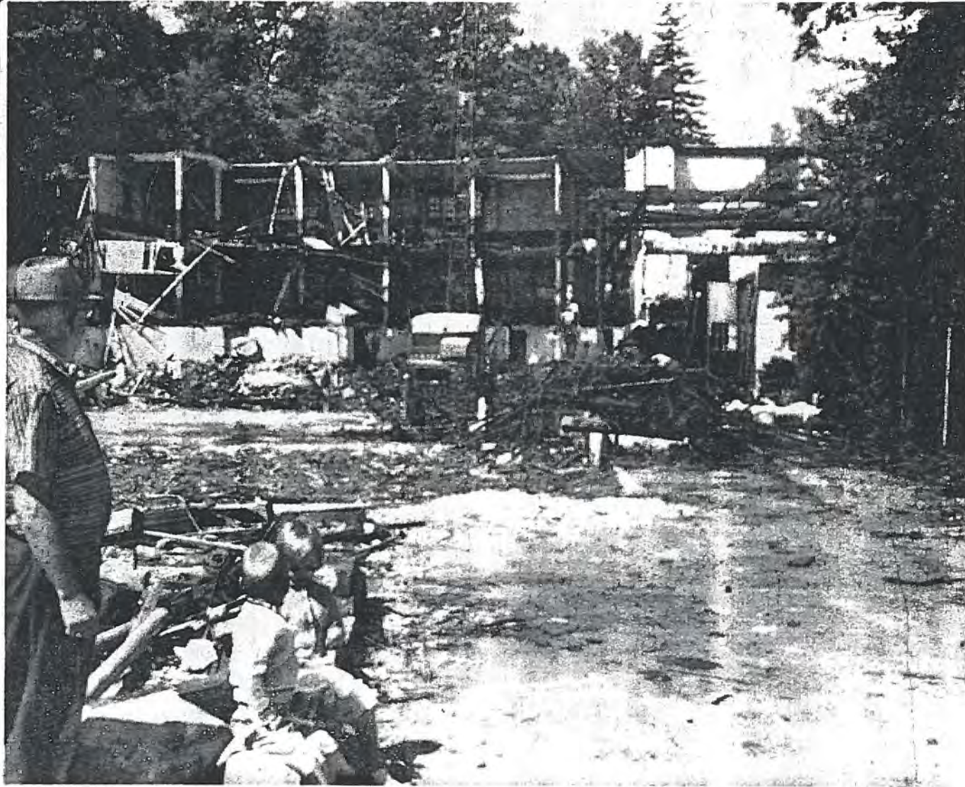
REMAINS OF HAT FACTORY of George McLachlan & Sons are inspected by Frank Ross and his grandchildren, Robert and Nadine Hallock. View
