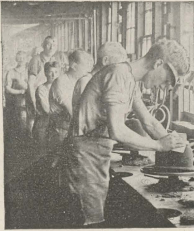
"FINISHING" OR SURFACING THE HATS
