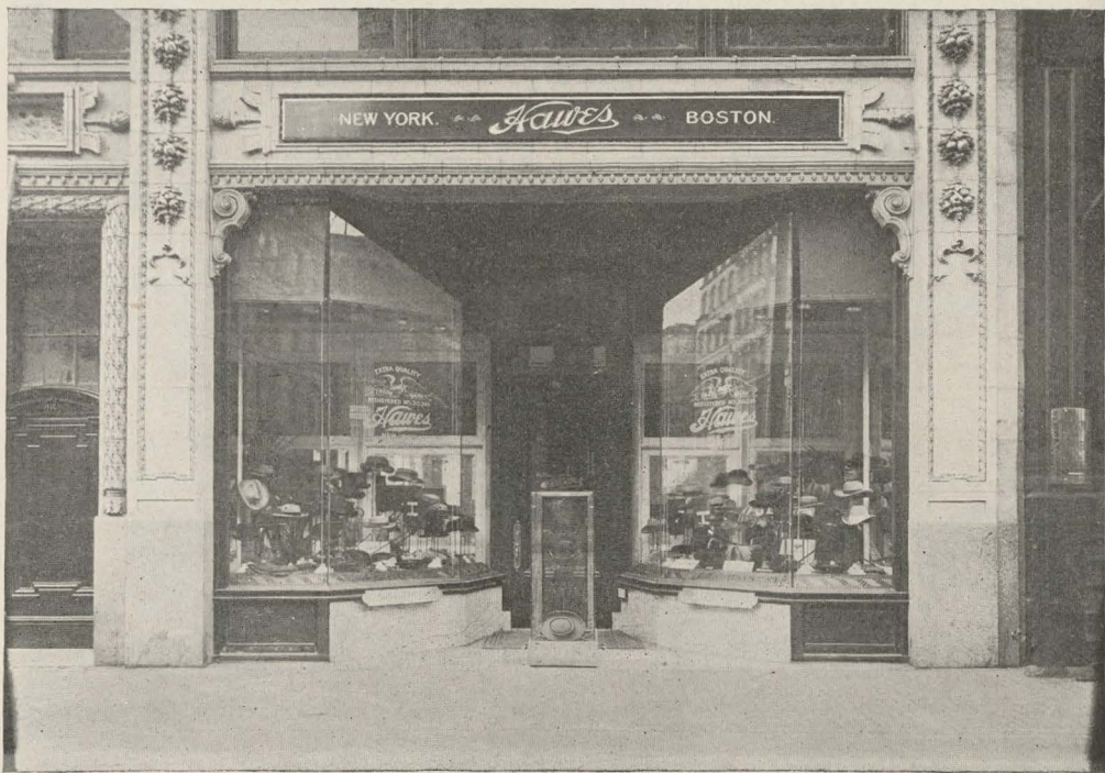
THE COMPANY'S BOSTON SALESROOMS AT 75 SUMMER STREET
