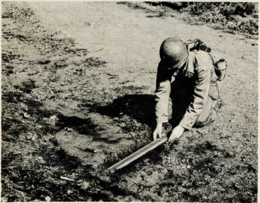
Figure 15. Installing yardstick mine on road shoulder.
