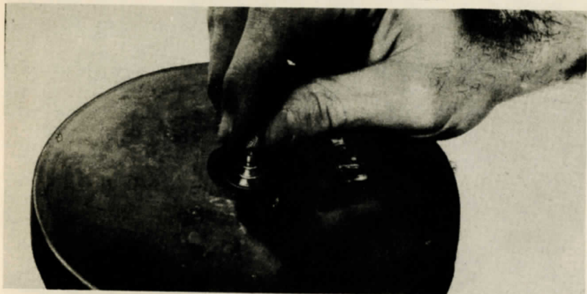
② Screwing safety cap into top of fuze.
